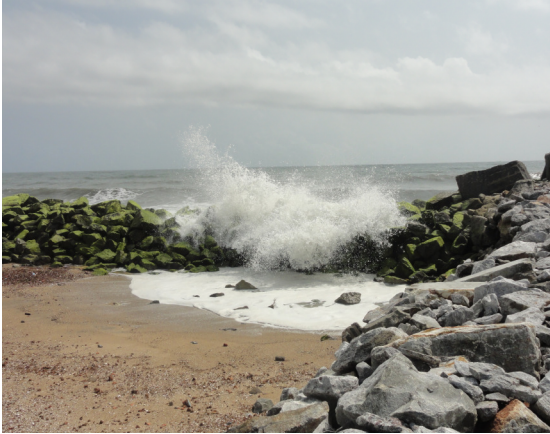
Fig. 1.2. Wave overtopping over coastline
