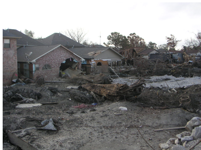
Fig. 1. Flow-related damage immediately landward of the 17th Street Canal breach site. In addition to the structural damage, trees were uprooted.
