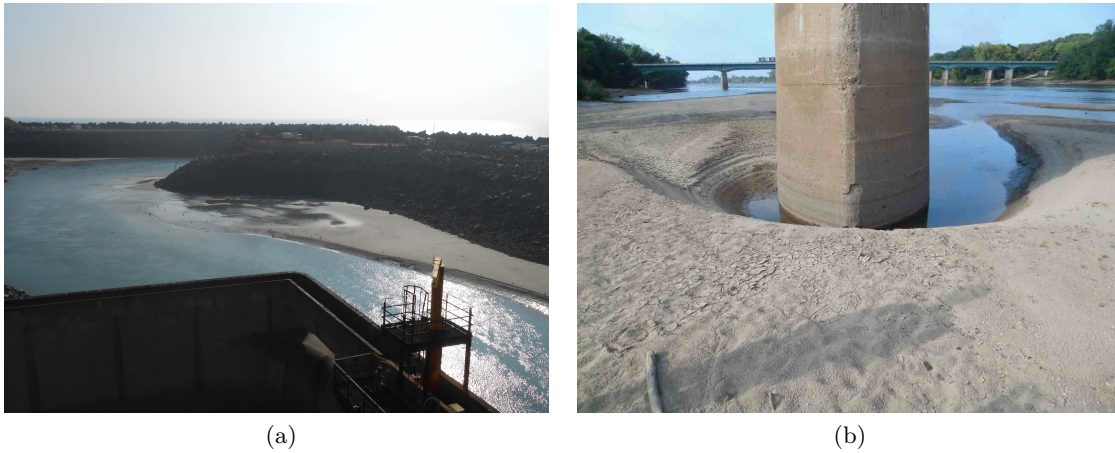
Figure 1: (a) Silting-up at the Flamanville cooling water intake (Credit: EDF). (b) Bridge scour photography (Credit: Public Domain Images – USGS [4]).
