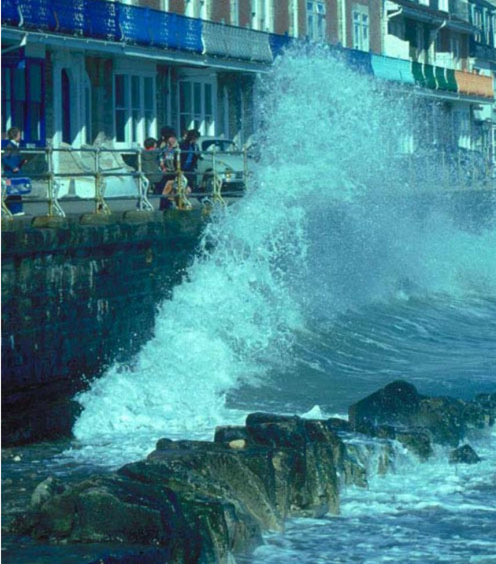
Figure 1.2: Snapshot of a wave impacting a vertical wall (photograph D.H.Peregrine).
