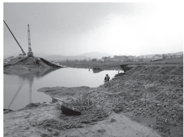
Fig. 1. River levee failure (Maruyama River, Japan, 2004)
